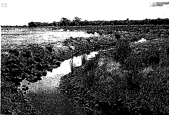
94. BEERMULLAH, WA, AUSTRALIA. An interceptor has prevented soil collapse by flooding (note rushes on upslope side), thus protecting crop below the bank. Spike rush ( Juncus ) is another indicator of imminent soil collapse, surface flooding, and anaerobic soils. Subsoils are dry, cemented, or subject to groundwater rising.
